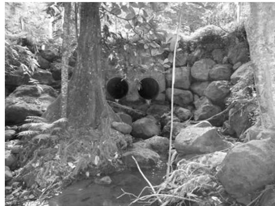
FIG 3. Photographs looking upstream at the open bridge (left) and the culverted bridge (right). The bridges serve as potential barriers to amphidromous organisms such as *Sicyopterus pugnans*, *Sicyopterus lagocephalus*, and *Stiphodon elegans*. The open bridge was identified as an easy barrier, while the culverted bridge was considered difficult to cross.
